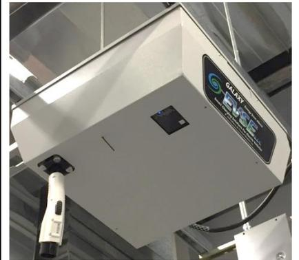
The Model 3722 electric vehicle charger provides 208 - 240V AC up to 30A. Designed as per the SAE J1772 requirements to meet or exceed all safety codes specified by UL and NEC, the unit is engineered for mounting overhead in public or private parking garages, while meeting or exceeding NEMA 3R specifications.
